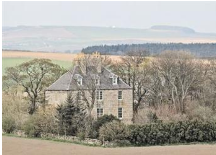
Figure 29: Picture of the 'modern' Rannieston House
